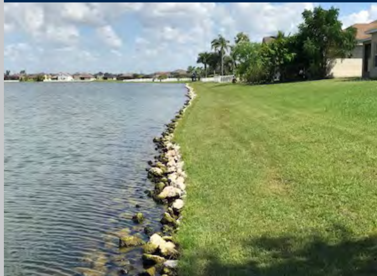
Pond Bank Restoration at Mira Lago CDD
