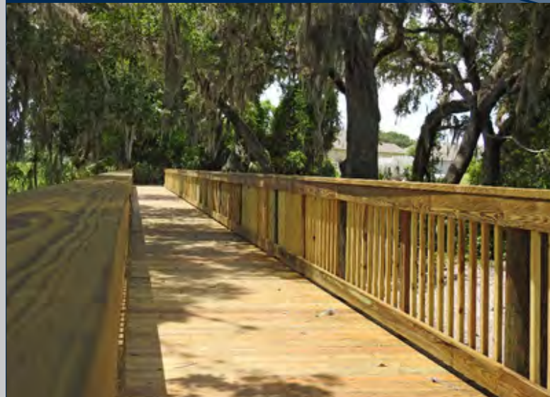
Pedestrian Boardwalk at Oak Creek CDD
