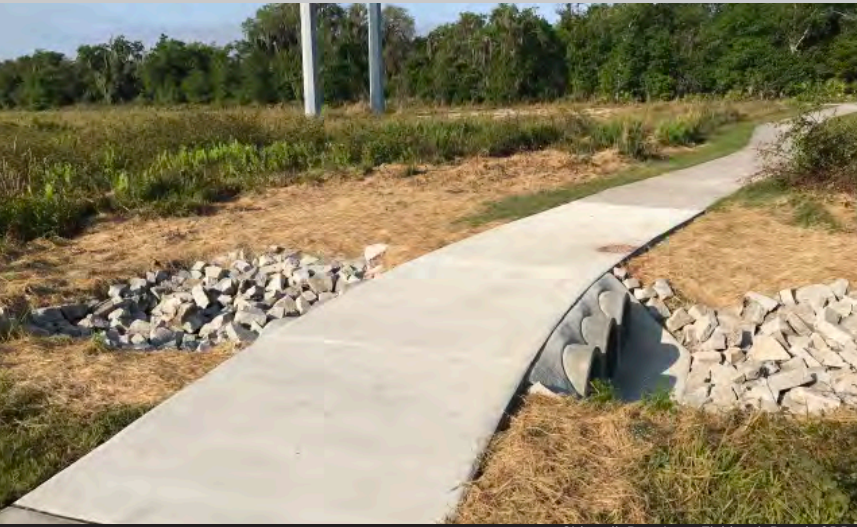
Sidewalk Repairs at Fishhawk Ranch CDD
