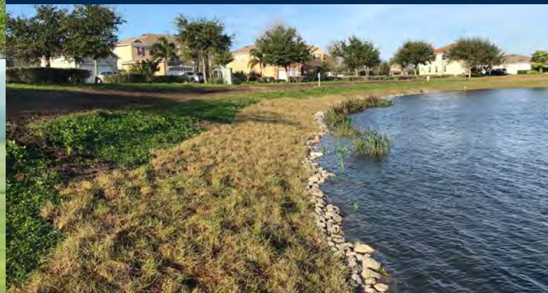
Pond Restoration at Harbour Isles CDD
